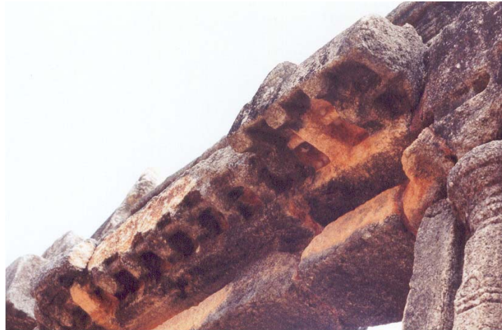
Plate 34. A close-up of the yantragala above the entrance to the Nalanda geḍigē. Photograph: courtesy P.J.J. de Bruijn.
