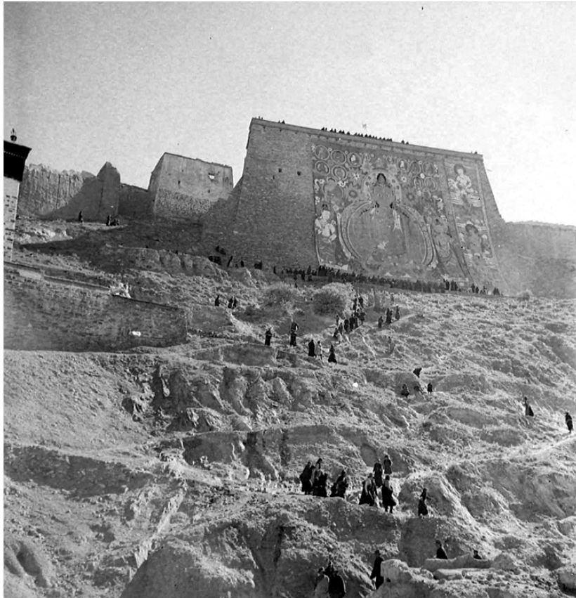
Figure 21: The pylon, built up against the mountain.
