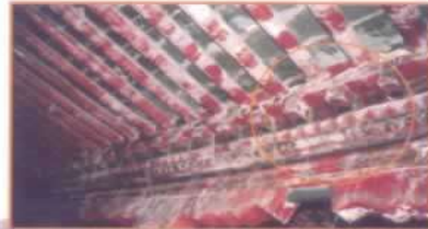
雨水从裂缝中溢出， 损坏屋顶的横梁。 Water Seeping into the cracks have damaged the roof beams.
