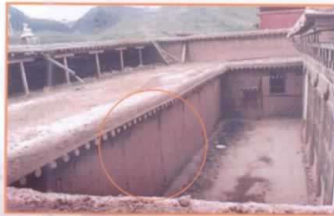
从屋顶的顶端往下看，大殿墙壁的裂缝清晰可见 Looking down from the roof-top, you can see the cracks in the walls of the hall.
