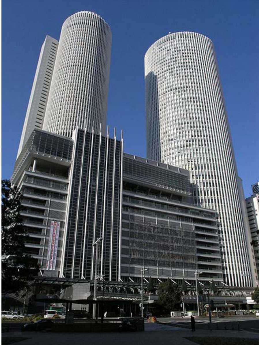
JR Central Towers in Nagoya, Aichi, Built in 1999
