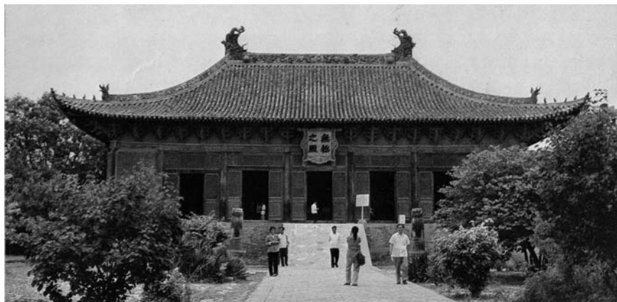
Fig. 85. Pavilion of the Three Clarities (Sanqing dian 三清殿). Yongle gong (Palace of Eternal Joy).
