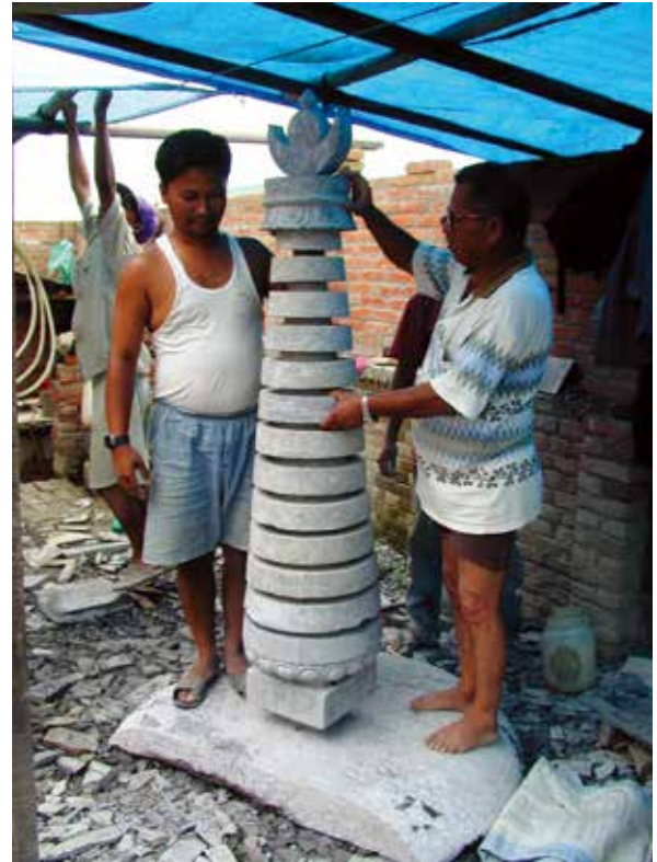
Figure 4. Nepalese stonemasons checking the fit of pre-carved components for the uppermost section of the stupa in Kathmandu, Nepal. Photograph by Holm Triesch, 2003.
