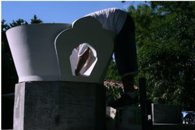
Drilling for installation.
