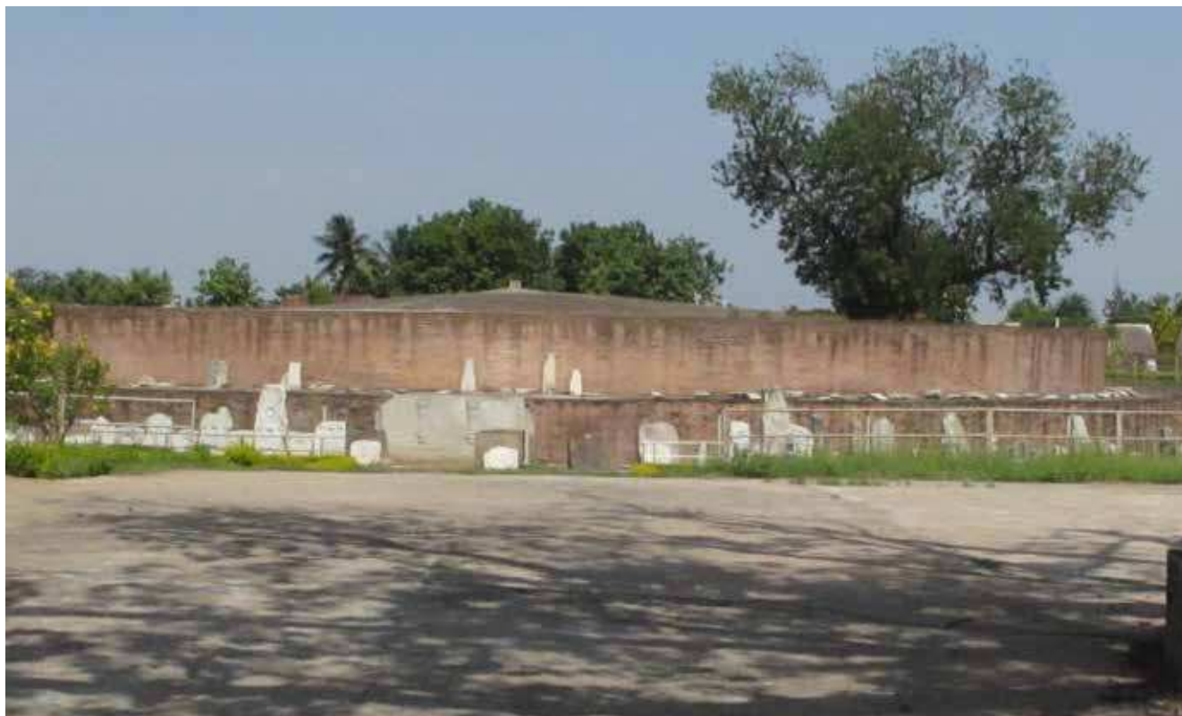
Figure 3 The Amaravati stūpa from the east, 2011
